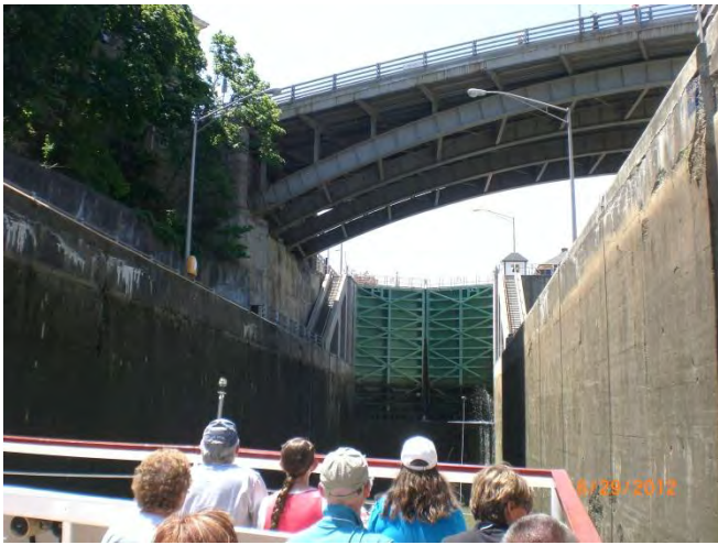
Entering the Lock
